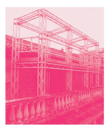
Square section aluminium truss with 25 cm long sides.
